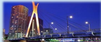
Chuo Ohashi Bridge
